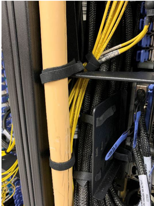
Figure 55.1: Zoomed Image of Routing Fiber Cables
