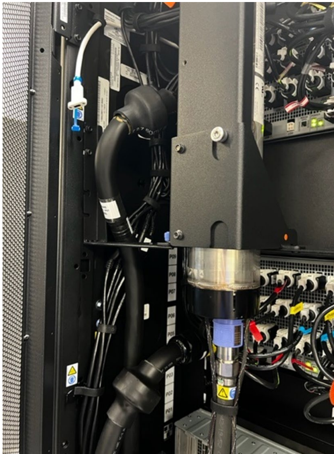
Figure 2: Line Cord Being Routed Under Reservoir Bracket
