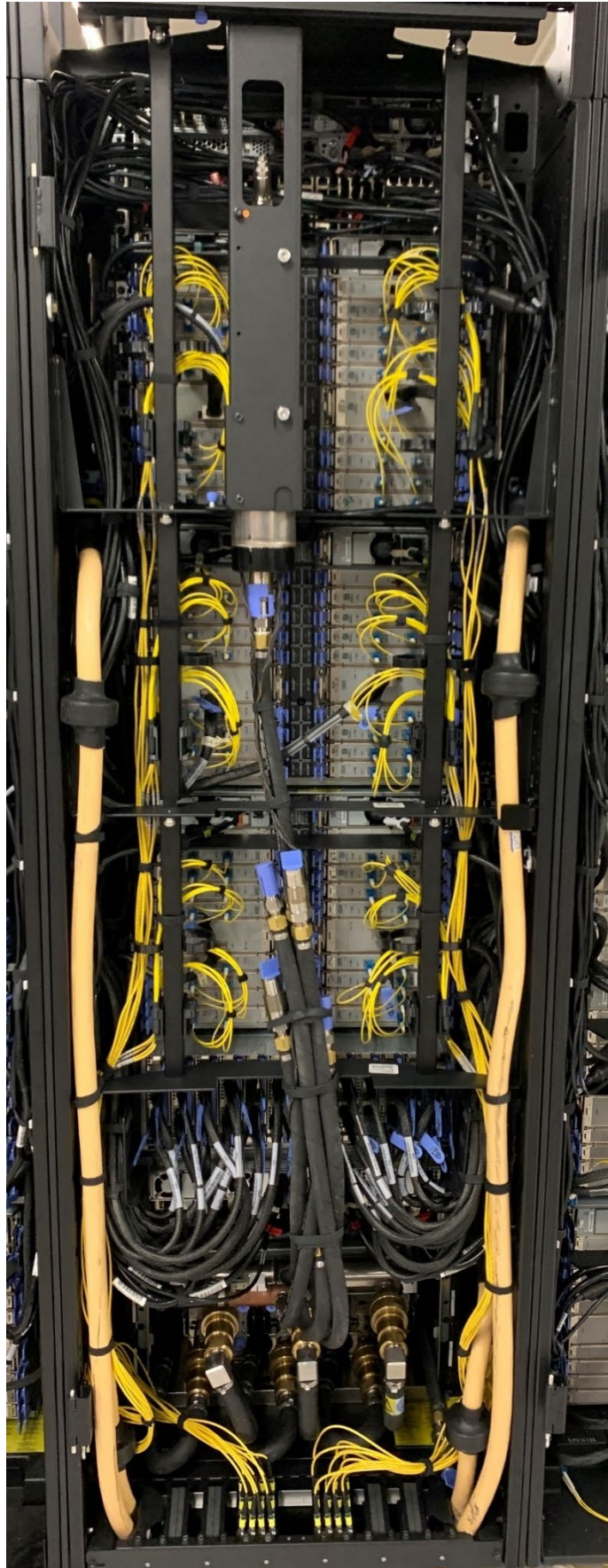
Figure 55: Routing Fiber Cables
