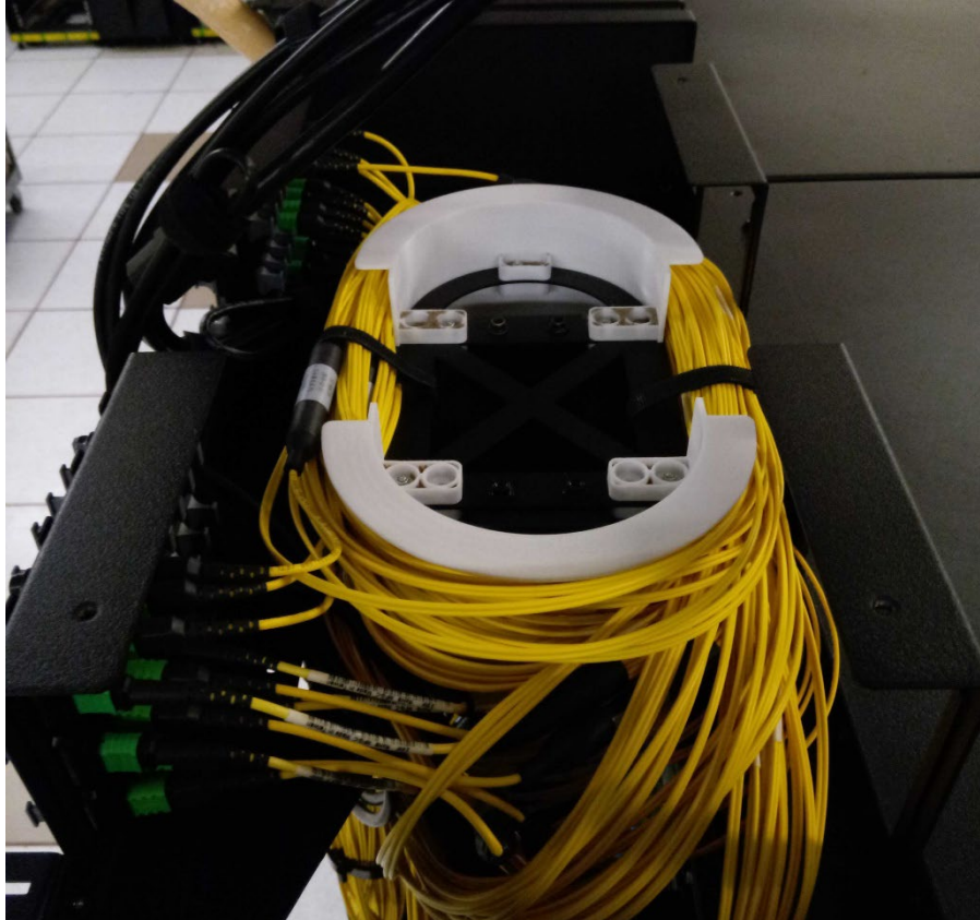
Figure 54: Fiber Cables in Top Exit Cabling Enclosure Including Integrated Cabling Spool
